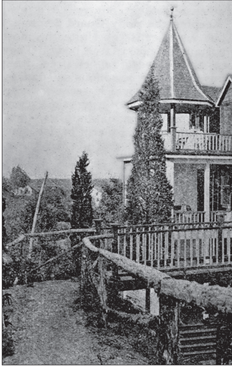
Observational tower in newly erected buildings at the Butler Yungborn.
